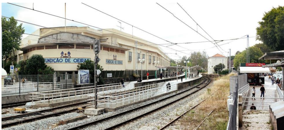
OEIRAS TRAIN STATION
