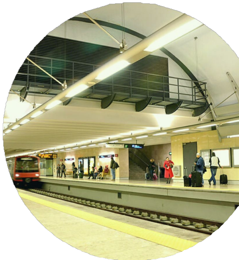
LISBON SUBWAY STATION
