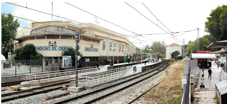
OEIRAS TRAIN STATION
